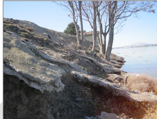
Figure 11. Area 1, with examples of Concrete Waste and Undercut Debris
